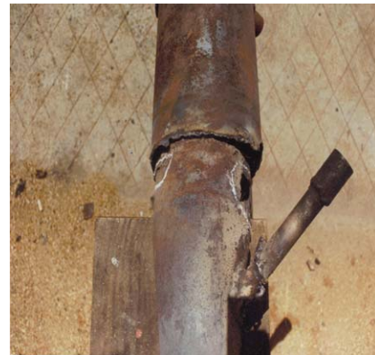
Fig. 2—(a) Damaged part at the lower portion of Mark II gasifier.
